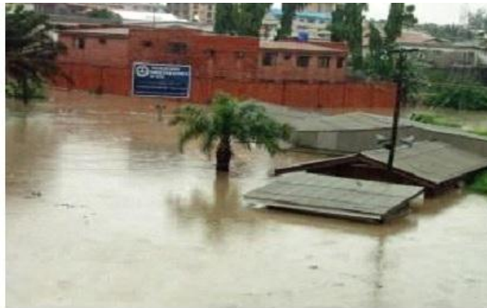
Figure 5. Flooded building in study area, 2019.
