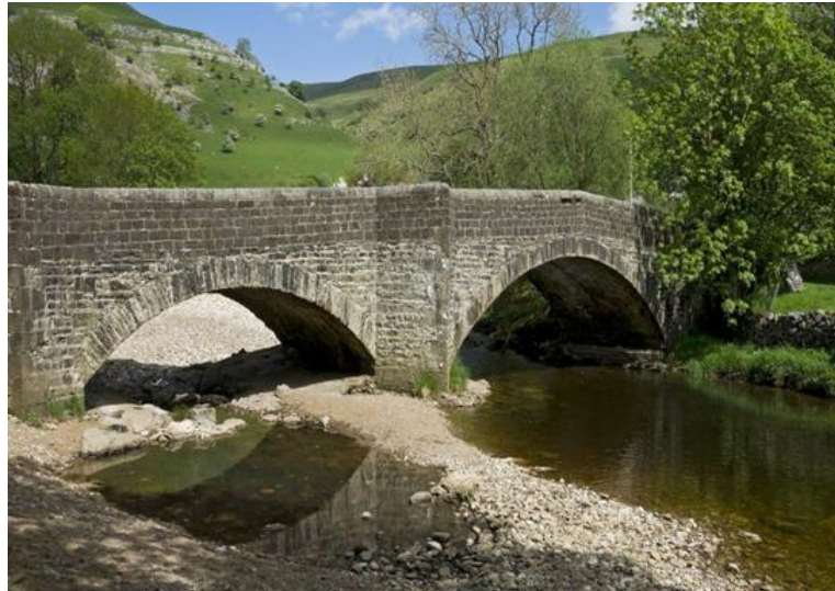
Figure 7. Yorkshire sewage spills into River Wharfe.
